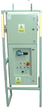
Switchgear type RKS5-1/5 is an electrical device designed for use in the underground mining pits in non-explosive conditions and on the ground.
